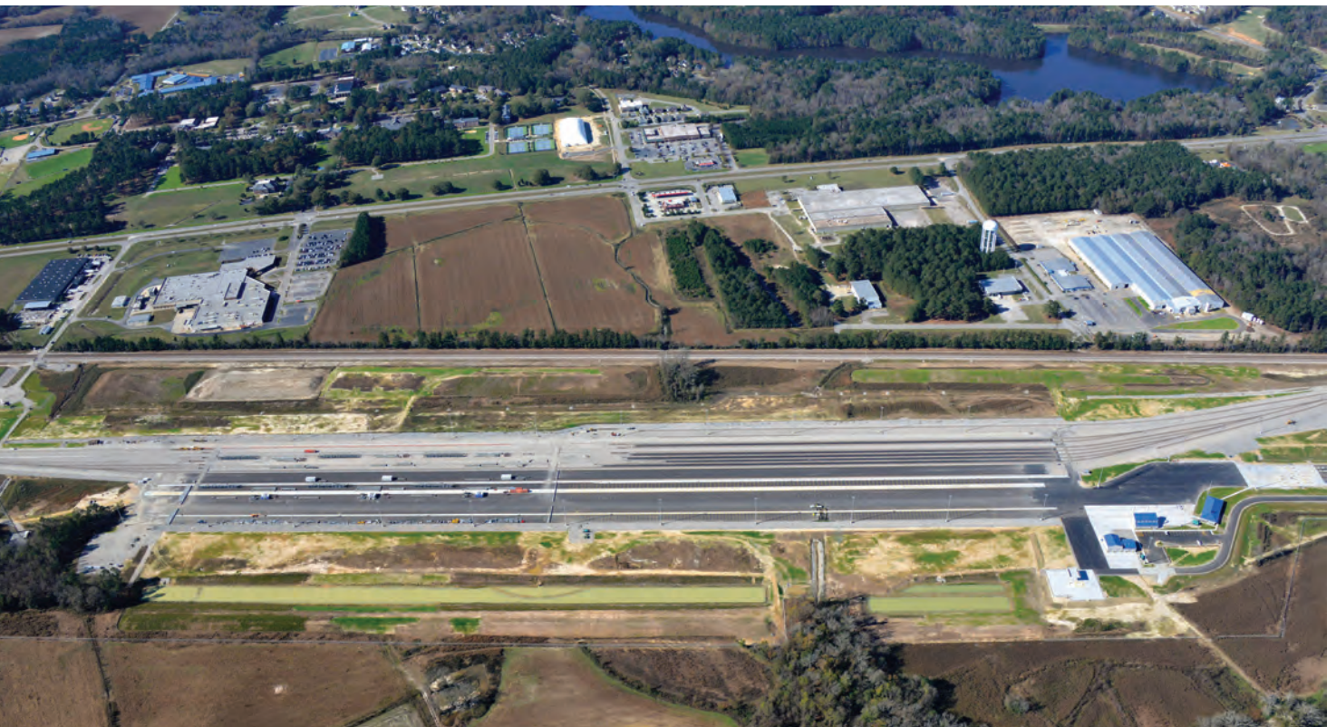
Terminal site looking west
